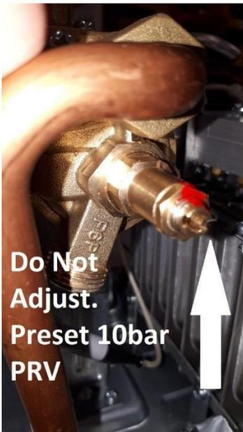
There is a safety valve on the side of the water control assembly set at 10bar. If the cold water supply pressure exceeds 10bar then this will pass water. Freezing conditions may also cause this to pass a small amount of water. Any adjustment of this valve will cause the valve to pass water at pressures lower than 10 bar and could damage furniture local to the heater.
