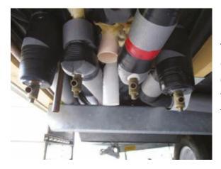
The above photo shows the plumbing under a home directly under a combination boiler. The two outer drain cocks are for the sealed central heating system and the two inner drain cocks are for the fresh water. Only open those for fresh water.
