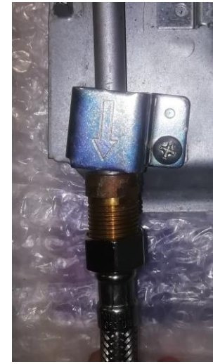
3. Fit the hot water pipe to the brass racord
