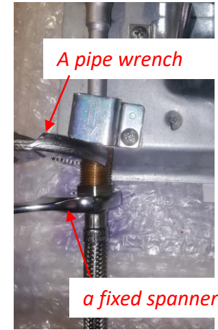
4. Tighten the brass racord and 19mm nut, using a pipe wrench and a 19mm spanner
