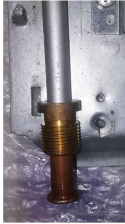
1. Fit the Heat Exchanger onto the Water Heater
