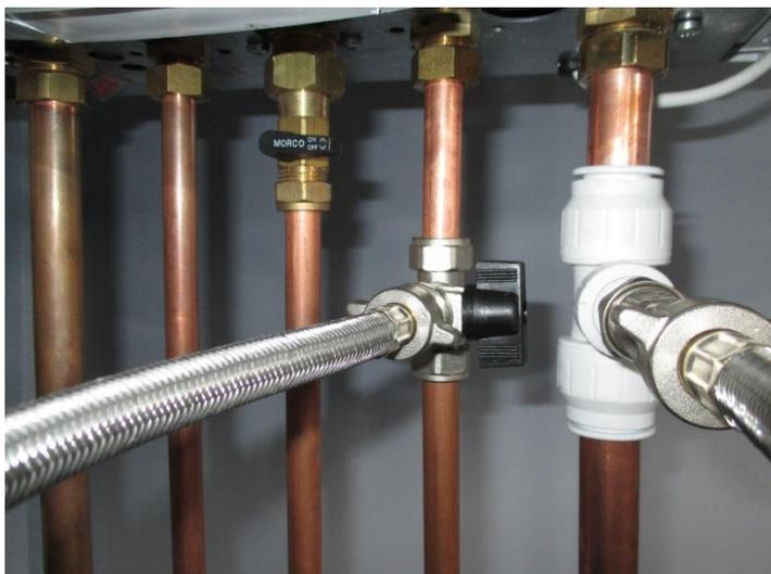
This is a photo of the underneath of a typical combi boiler before the gauge is fitted with the filling loop in place. The 15mm copper pipe 2<sup>nd</sup> from the right is the cold water inlet.
