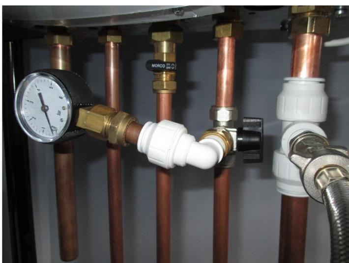
This shows a pressure gauge fitted to the cold water inlet pipe connected via the filling loop tee. Open the black plastic tap and the gauge will read the “standing pressure”. To read the “operating pressure”, open each hot outlet in turn and take a reading from the gauge while the hot water is running. This will provide you with the “operating pressure” for each hot outlet. The connection on the filling loop tee is 1/2inch BSP.
