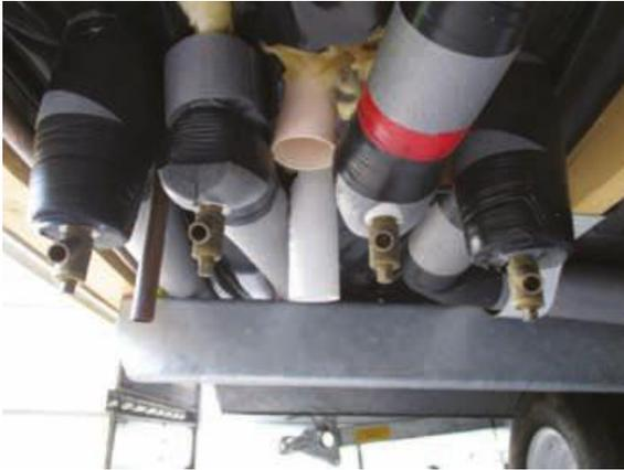
The above photo shows the plumbing under a home directly under a combination boiler. The two outer drain cocks are for the sealed central heating system and the two inner drain cocks are for the fresh water. Only open those for fresh water.
